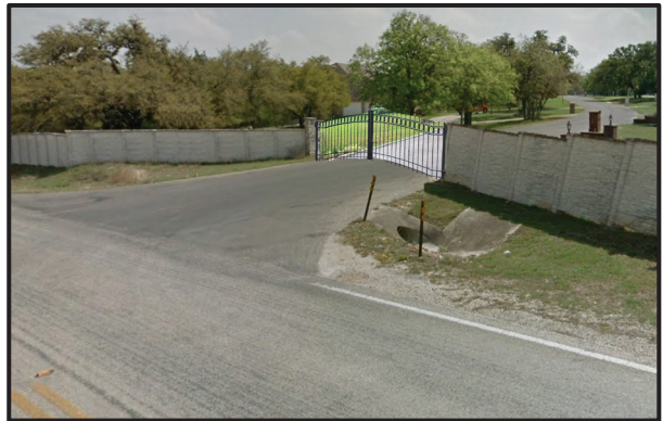
Figure 21 – Emergency Access Gate
