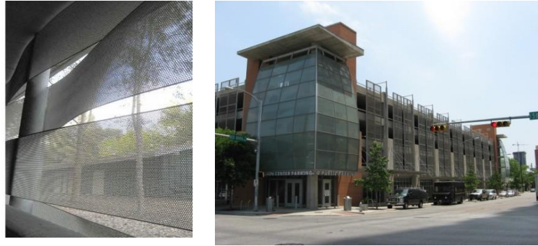
Figures 7-13 Illustrative Examples of Parking Garage Screening
