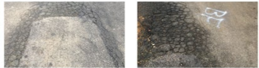
Pavement Condition 0 - 10 (Failed)
