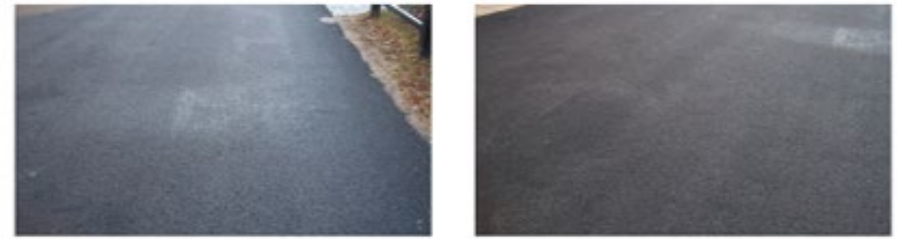
Pavement Condition 71 - 85 (Satisfactory)
