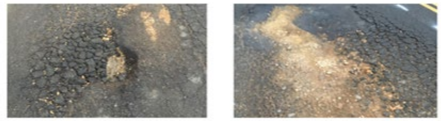
Pavement Condition 0 - 10 (Failed)
