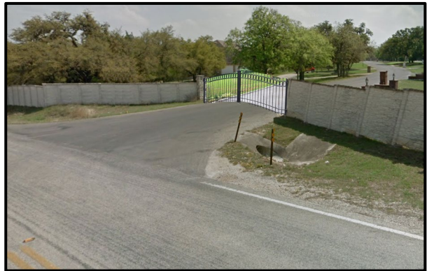
Figure 21 – Emergency Access Gate
