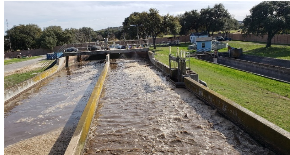
Extended aeration basin at existing WWTP
