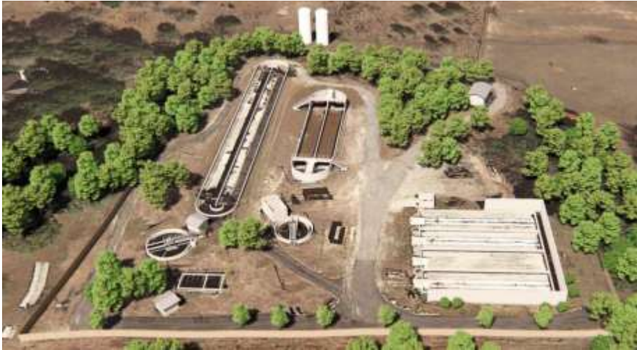
Aerial view of existing WWTP
