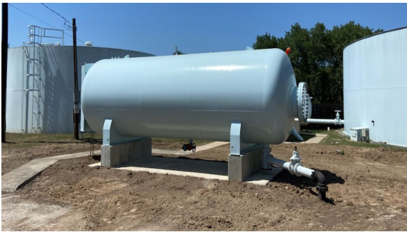
New 9000 gallon hydropneumatic tank and ribbon cutting photo.
