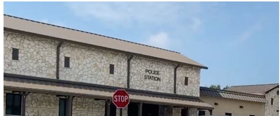
Existing Metal Roofs
