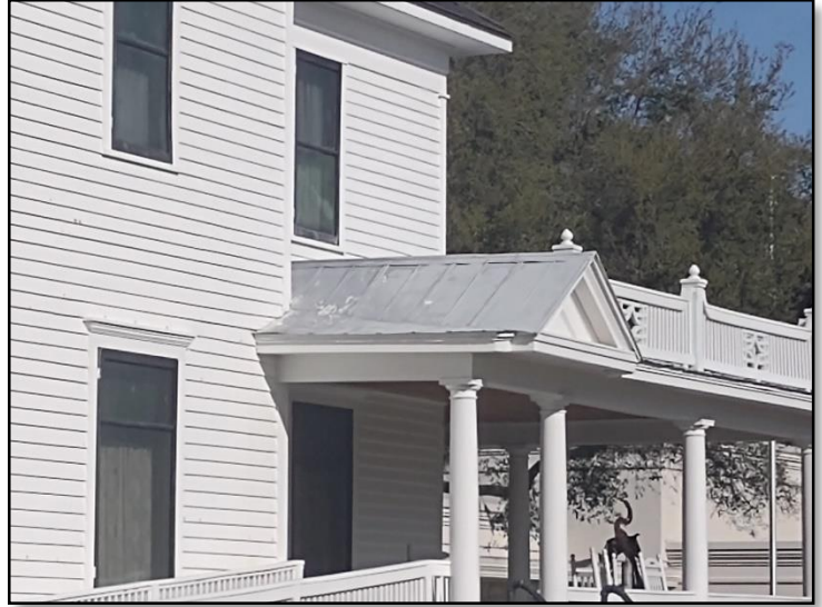
The front porch roof is metal built on 1911
