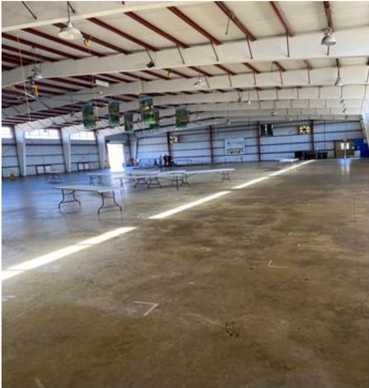
LEHMANN POLK EXPO BUILDING BAY
