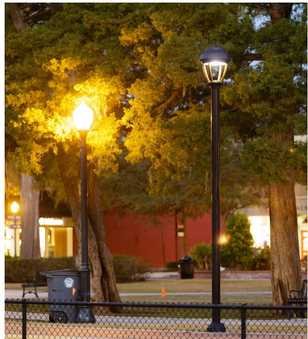
The photo depicts prohibited unshielded pedestrian walkway lighting versus fully-shielded lighting installed with 2700K CCT LED light.
