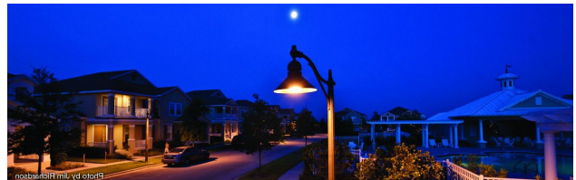
Dark-Sky compliant street light. The fixture is fully-shielded and downward facing with a warm color temperature.
