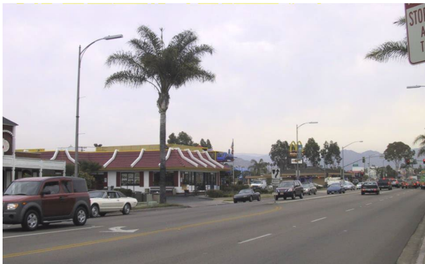
Mid-block left turn lanes, which facilitate access to individual businesses, may impede traffic flow
