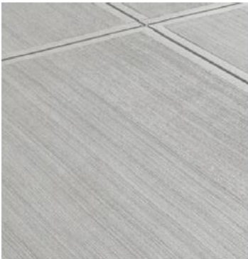
Concrete Flatwork broom finish
