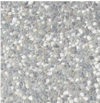
Concrete Flatwork heavy aggregate finish
