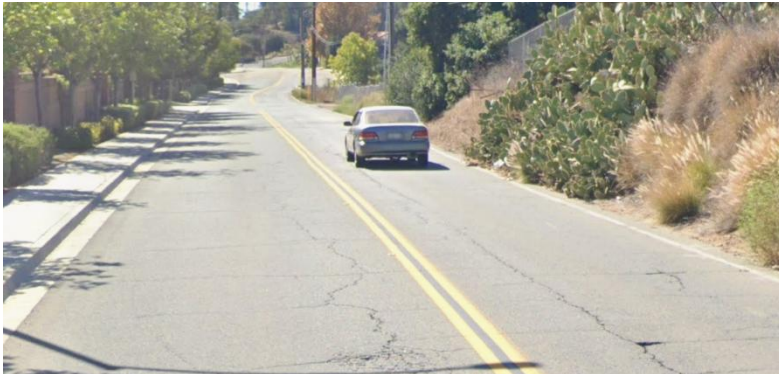
Existing Street Conditions on North Iris Lane
