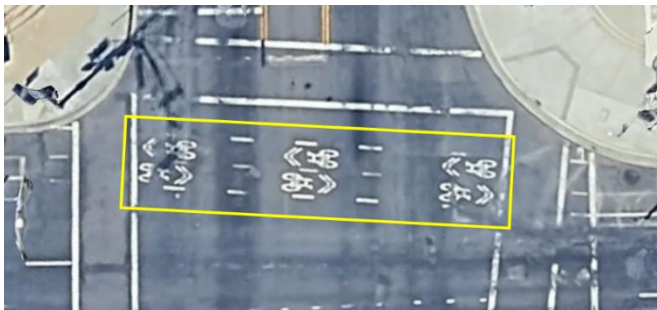
Existing Conflict Striping in Class IV Facility (Aerial View)
