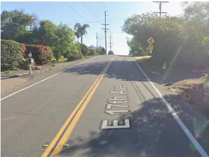
Existing Conditions on East 17 th Avenue
