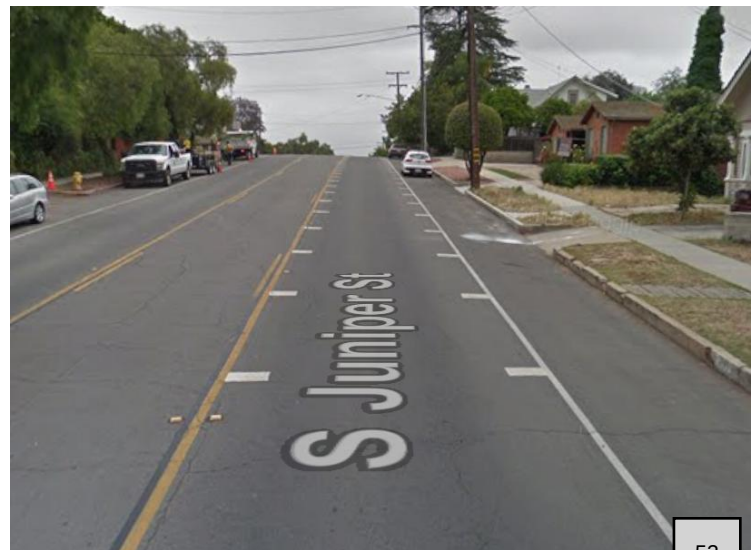
Speed Reduction Markings – South Juniper Street
