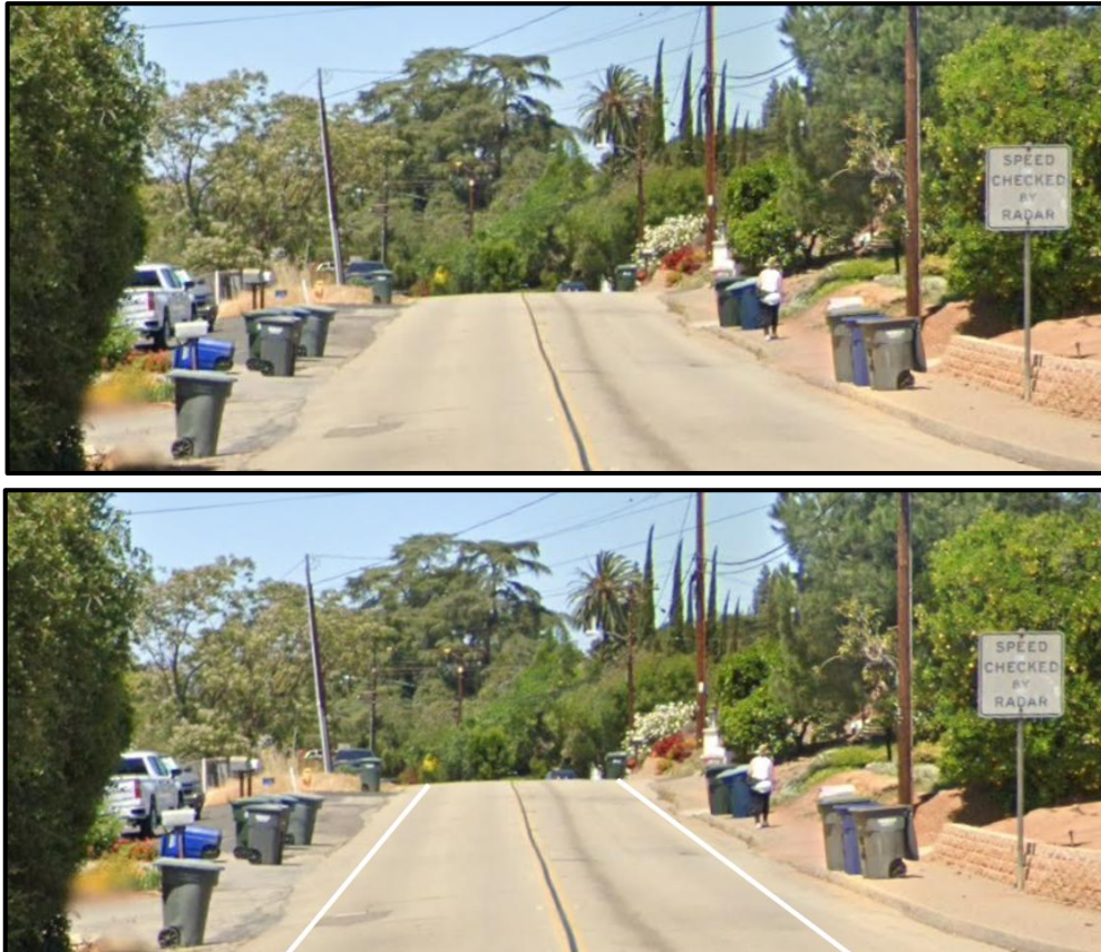
Figure 12. Before and After Edge Line Striping on Juniper Street.
