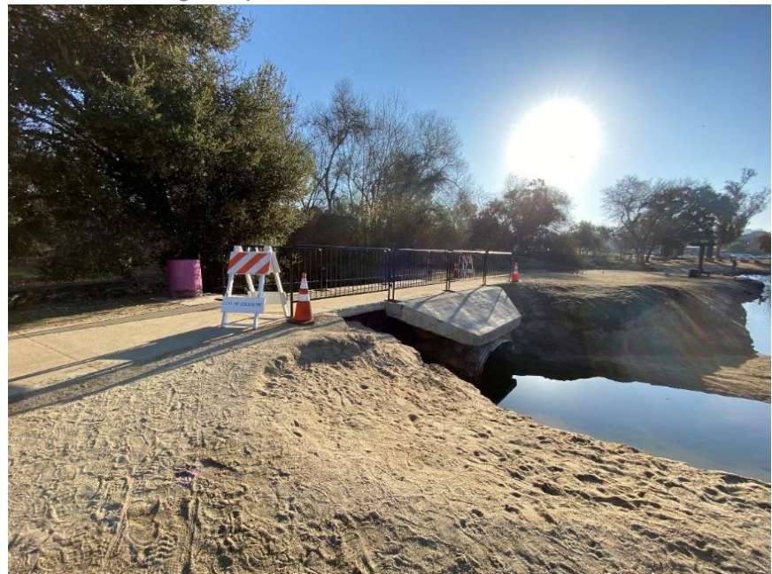
Kit Carson Bridge Repair
