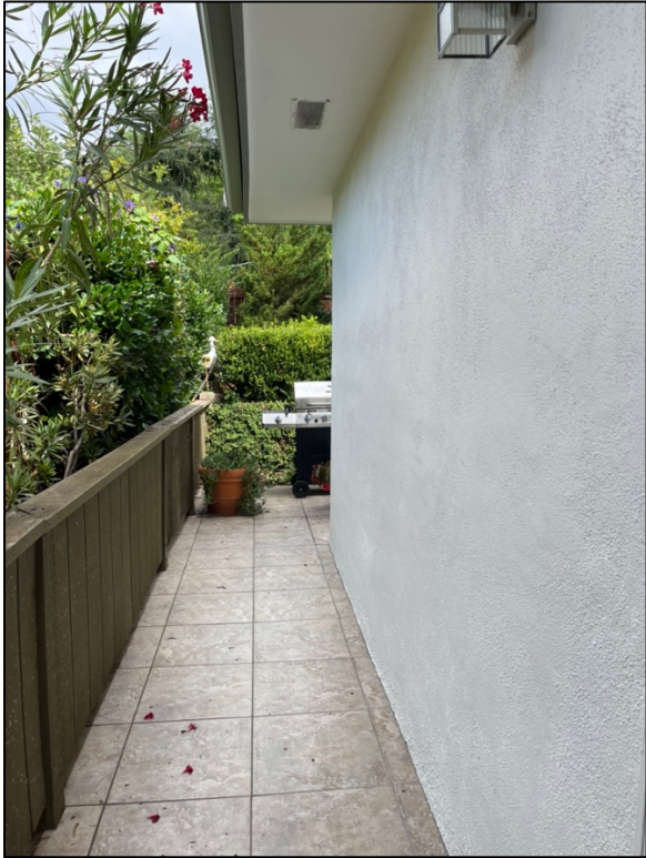
View of northerly side of house, through side gate (looking east)
