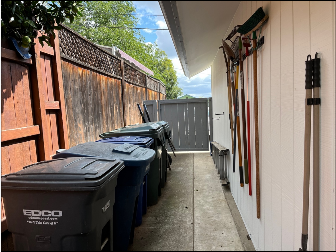
View of side of easterly side detached garage (looking south)
