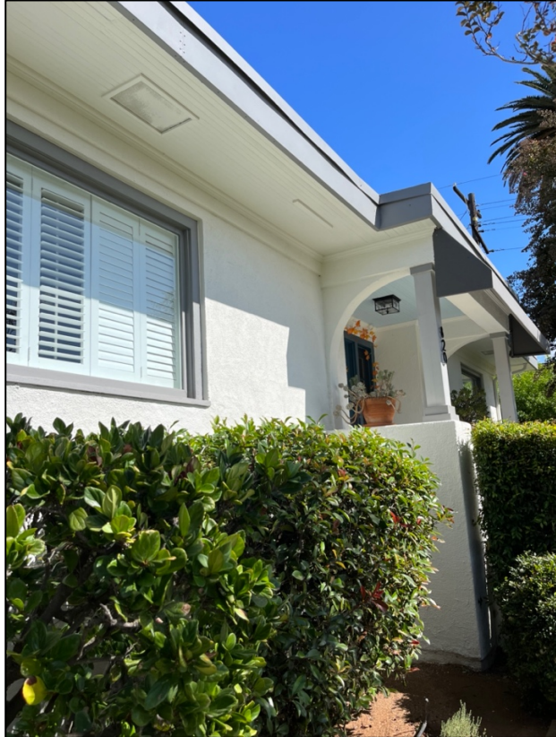
View of front stoop and northerly bay window (looking south)
