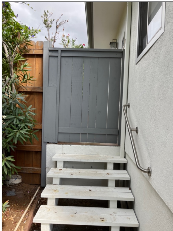
View of northerly side of house-side gate (looking east)
