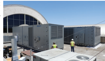
John Wayne Airport Air Handler Replacement Santa Ana, CA
