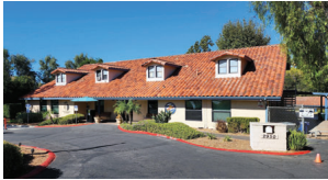
EXISTING ADMINISTRATION BUILDING
