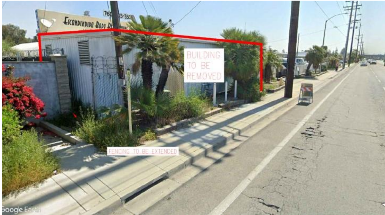
Looking northeast along W. Mission Road
