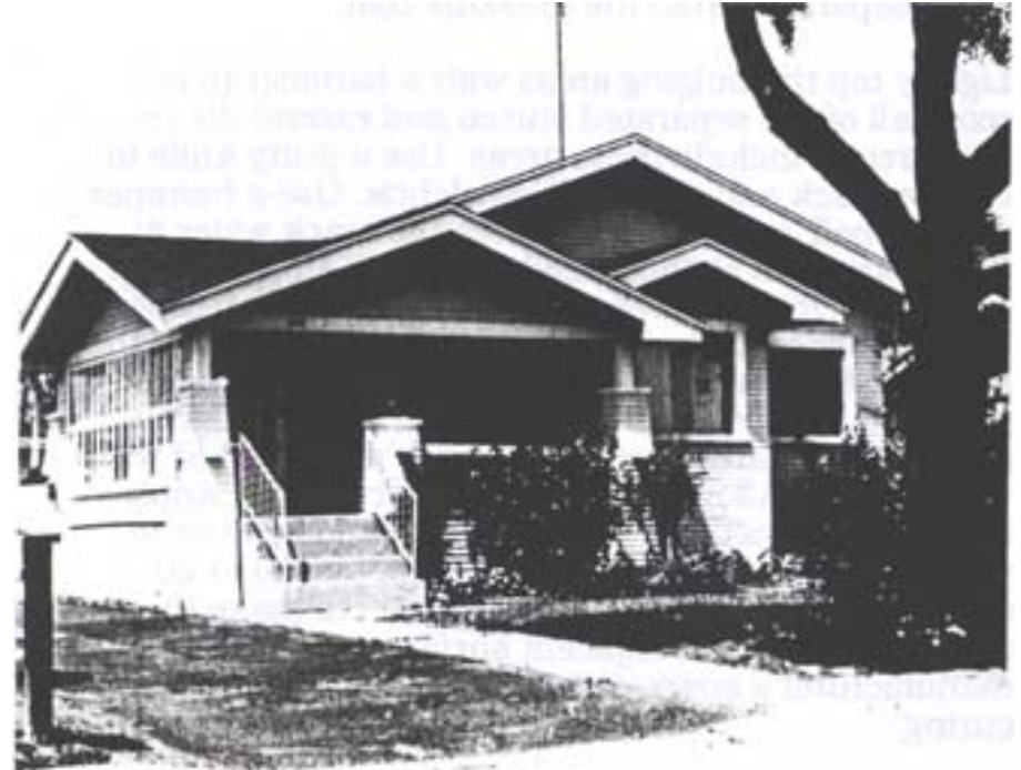
Metal handrails are not appropriate replacements and look out of scale.
