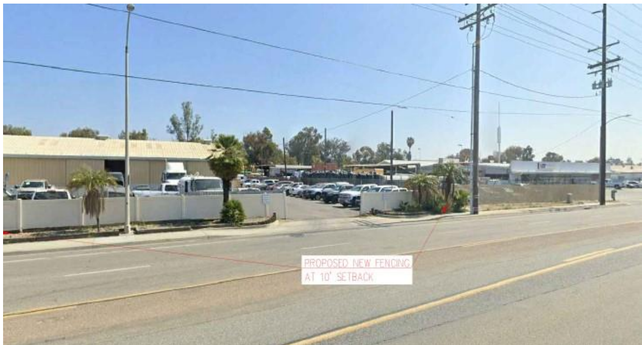
Looking southeast along W. Mission Road at secondary access
