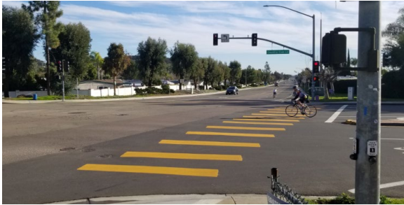
Broadway-Rincon Intersection Fully equipped with sidewalks and signals
