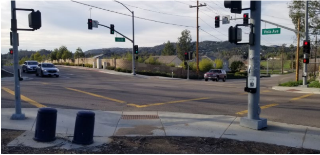
N. Ash – Vista Intersection Fully equipped with sidewalks and signals
