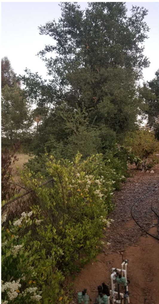
Figure 3c – Example of tree/shrub growth through the property line fence and proximity of sprinkler set to fence.
