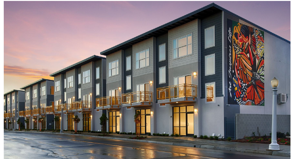
Example of live-work dwelling units
