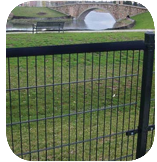
Four Foot High Fencing Proposed at the Top of the Channel to be Black Tubular Steel or Black Metal Wire Fencing with Top Rail
