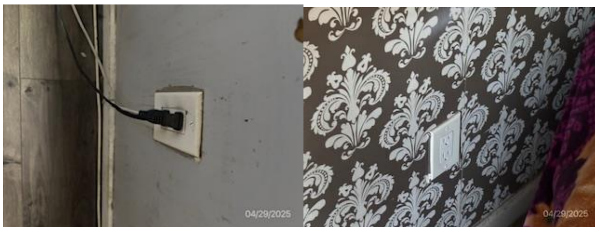
Item #10 Receptacles all have covers and no exposed wires.
