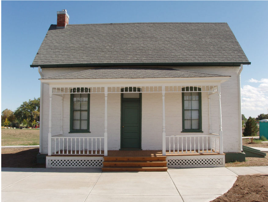
Photo 1 Southwest (main) Façade, camera facing northeast
