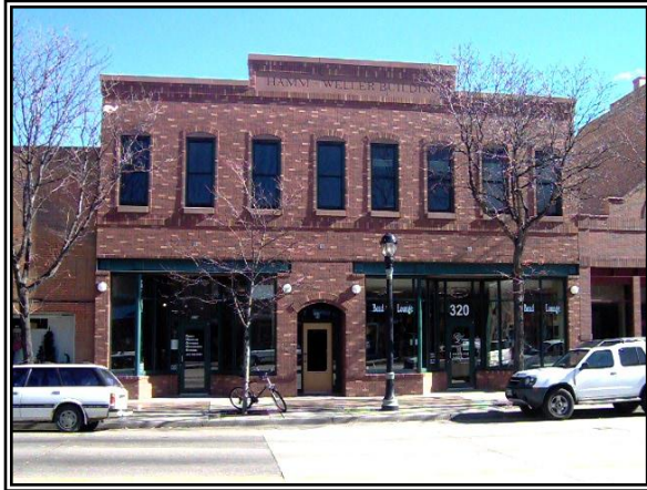
This new [~1990] building successfully complements an immediately proximate ~1890 building by use of multiple treatments: Street-orientation; use of kick-plates and extensive first floor windows; second-floor complementary windows w/sill and lintel features; arched/highlighted entry; use of brick; and parapet roof with inscription.
