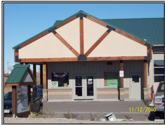
Use of heavy timbers to define entries, both small-scale and large-scale, is common throughout Colorado. Timbers and split-faced/colored concrete blocks complement one another. Covered entry feature adds interest and weather protection.
