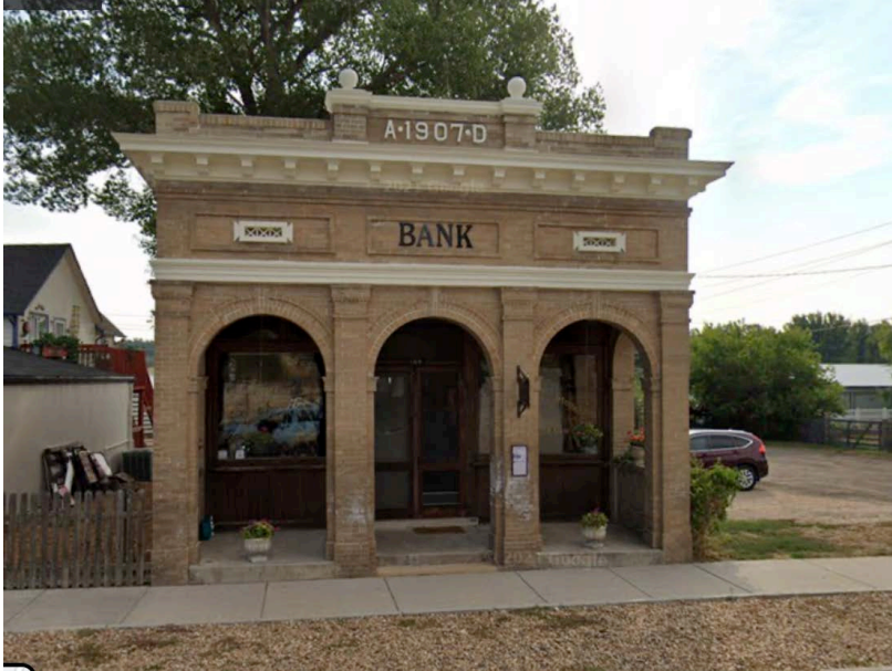
West (street-facing) primary facade Source: Google Maps, Street View (see additional pages for additional photographs)
