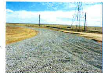
Photograph SCR-1. Stabilized construction roadway.
