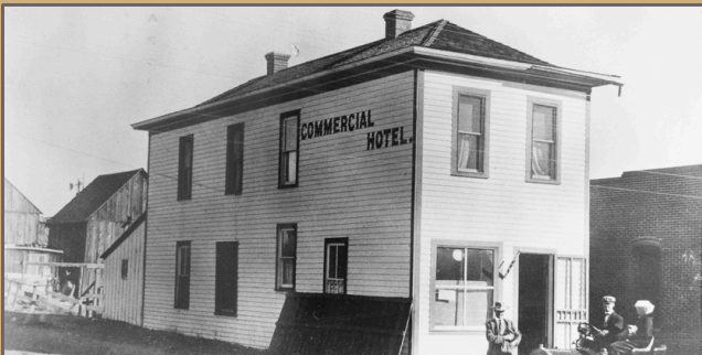
Commercial Hotel, Former Site to the West of 377 E Kiowa Avenue
