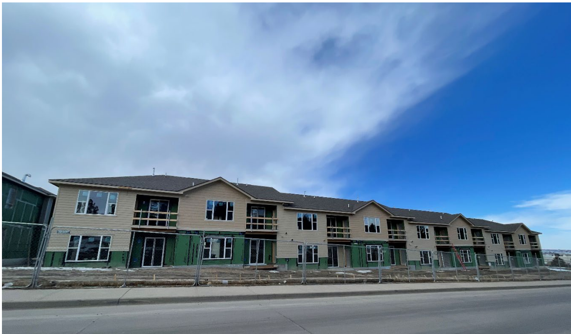
Current Site – (Under Development)
