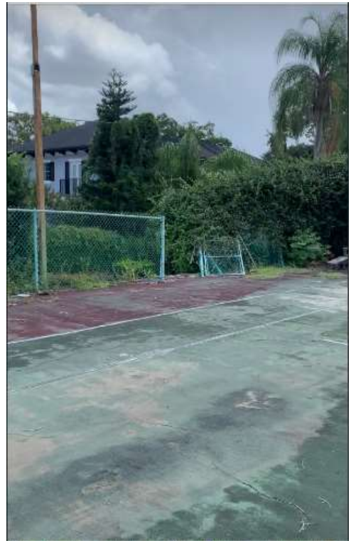
Looking at Southeast corner of court
