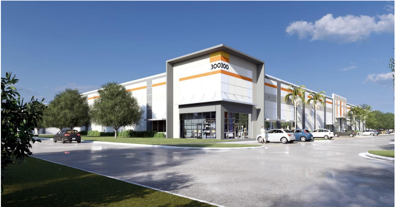
INTERNAL VIEW FROM NORTHWEST CORNER OF SITE
