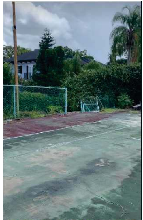
Looking at Southeast corner of court
