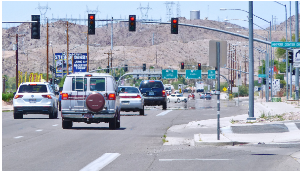
SR238 ROADWAY IMPROVEMENTS
