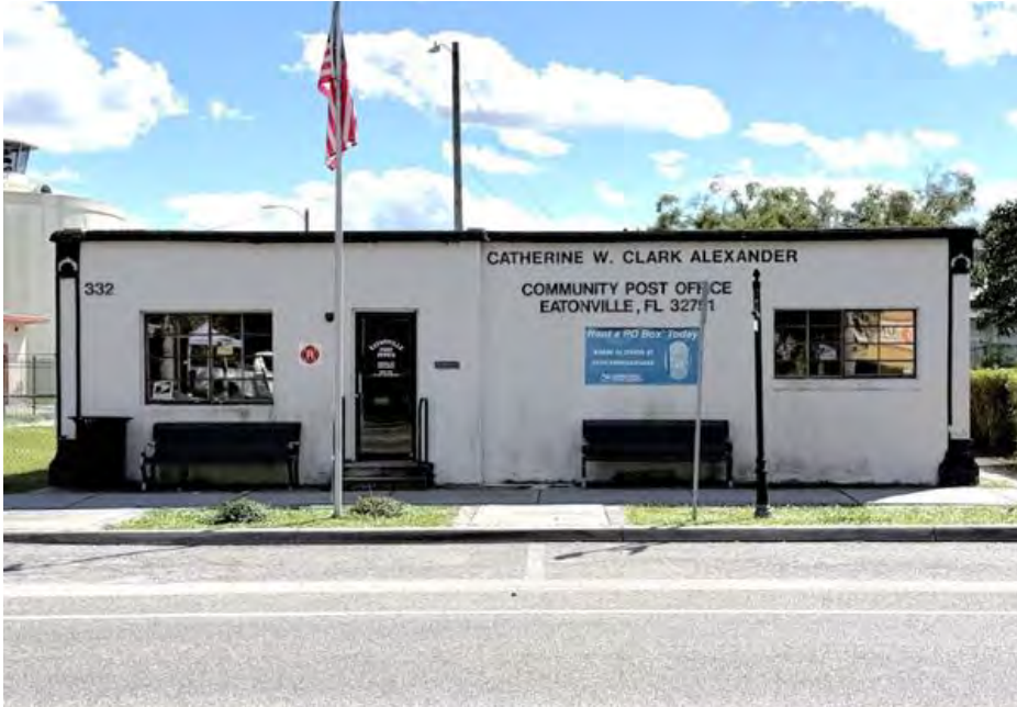
Community Post Office (Built 1959)
