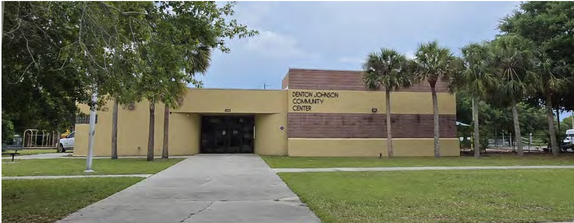
Denton Johnson Community Center
