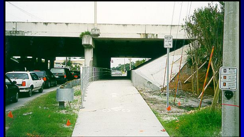
Pedestrian Access Under I-4
