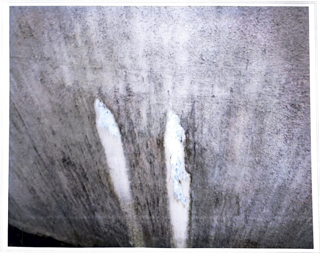
Staining and Cracking with Efflorescence on Exterior Wall
