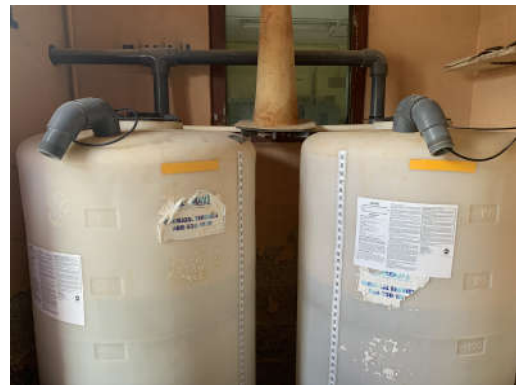
Photo 4-3: Chlorine Chemical Feed System
