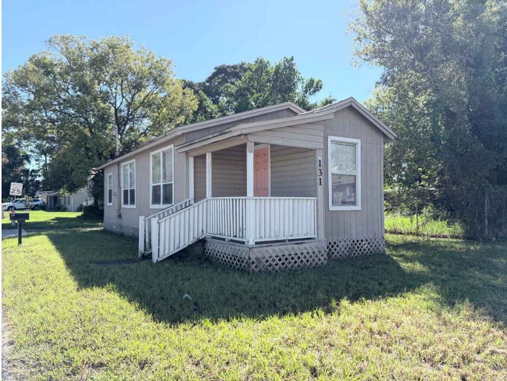
Figure 38: Frame vernacular style at 131 N. Wymore Road, 2025. | Planning 2 Preserve
