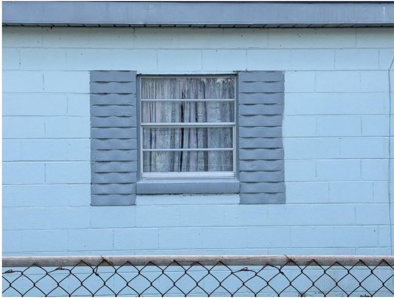
Figure 50. 10 Moseley Avenue with embedded shutters. | Planning 2 Preserve
