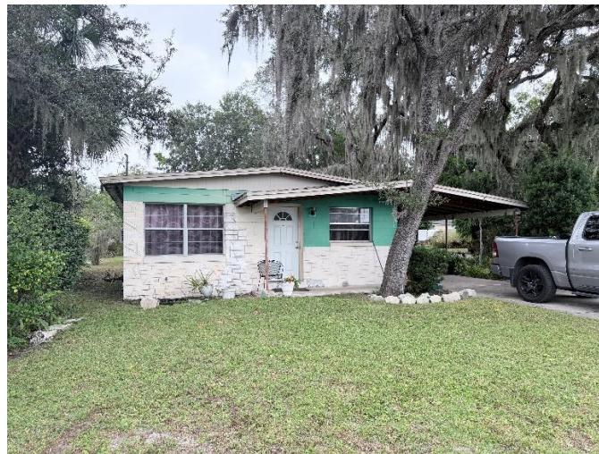
Figure 47. 32 Elizabeth Street with ashlar stone facing. | Planning 2 Preserve
