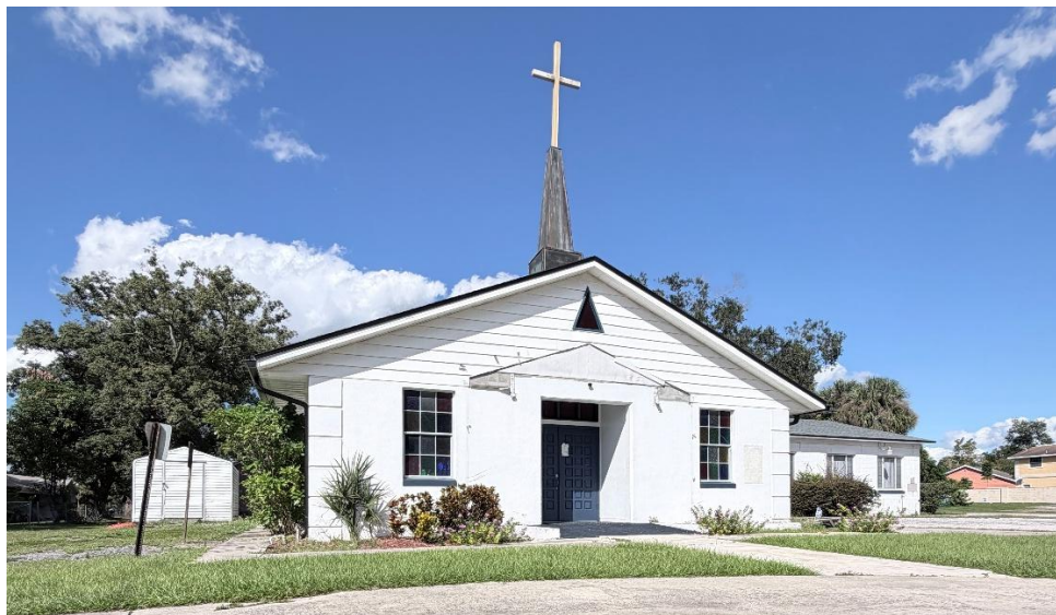
Figure 49. 549 E. Kennedy Blvd. with quoins at exterior corners. | Planning 2 Preserve
