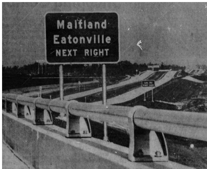
Figure 5. Recently completed Interstate 4 in the vicinity of Eatonville in 1965. | Orlando Sentinel
