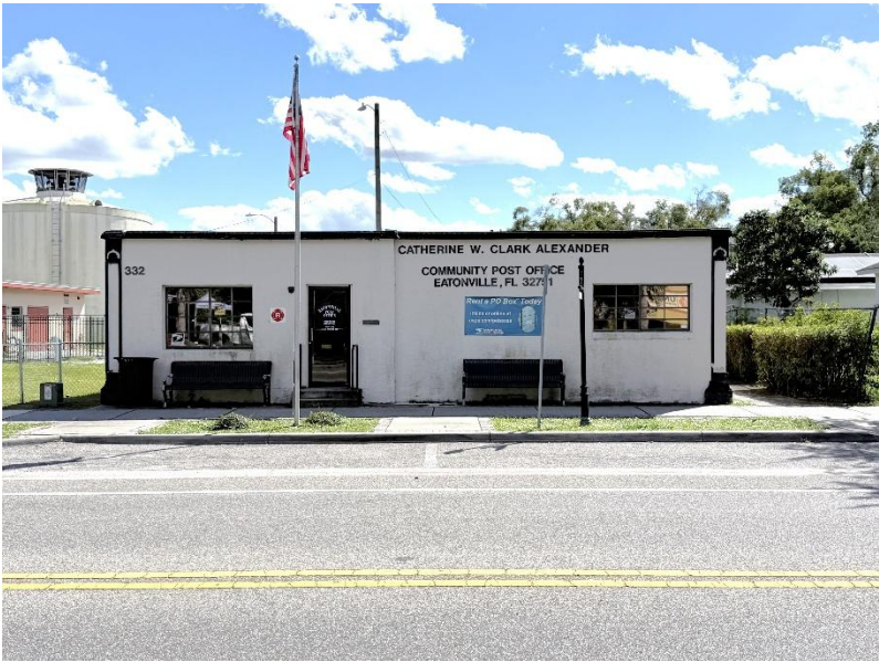
Figure 52. Community Post Office, 332 East Kennedy Boulevard. | Planning 2 Preserve
