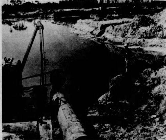
Hubbard Construction Co. employe Henry Adams stands on bank of future lake. Pump (foreground) will be removed when digging is completed and water allowed to fill the cavity.
