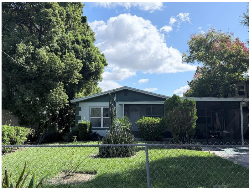
Figure 48. 175 Johnson Street with quoins at exterior corner. | Planning 2 Preserve
