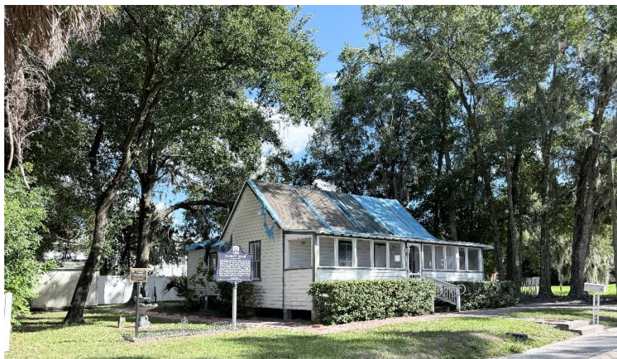
Figure 56. Moseley House, 11 Taylor Avenue. | Planning 2 Preserve
