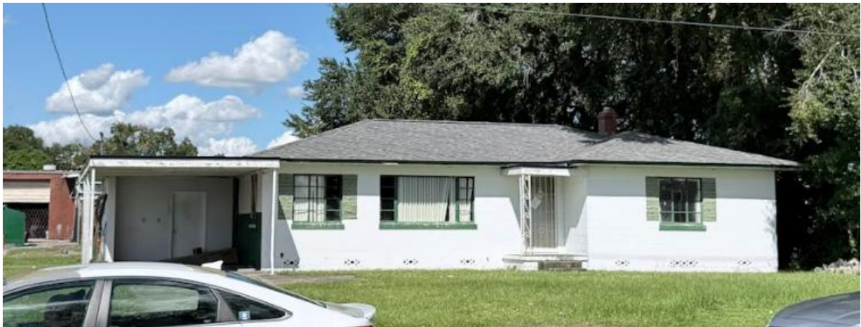
Figure 51. 15 E. Kennedy Blvd. with embedded shutters. | Planning 2 Preserve
