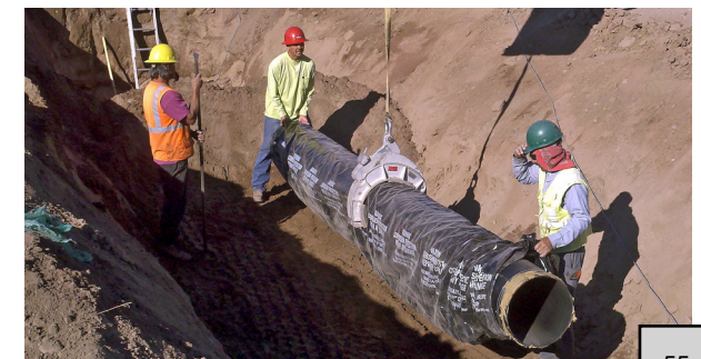
Town of Queen Creek – Water / Sewer On-Call Engineering Services
