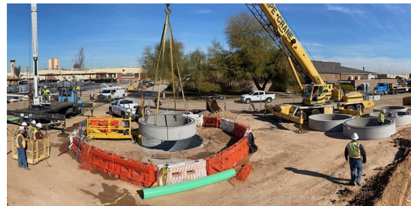
USACE – Luke Air Force Base, Sewer Lines / System Replacement
