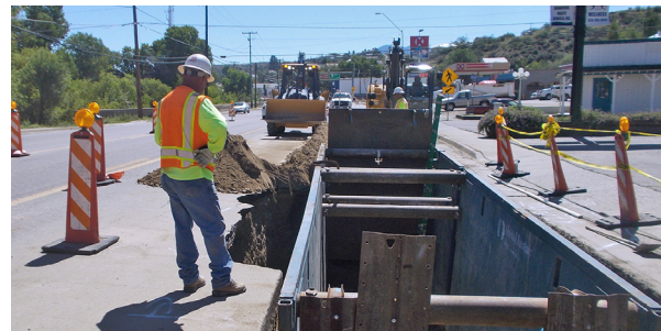
City of Globe – US 60 Water Main Replacement
