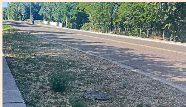
Town of Eagar – Main Street Sewer
