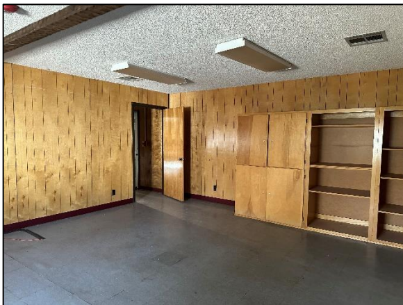
Interior View (Building C)
