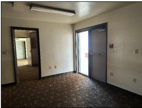
Interior View (Building A)
