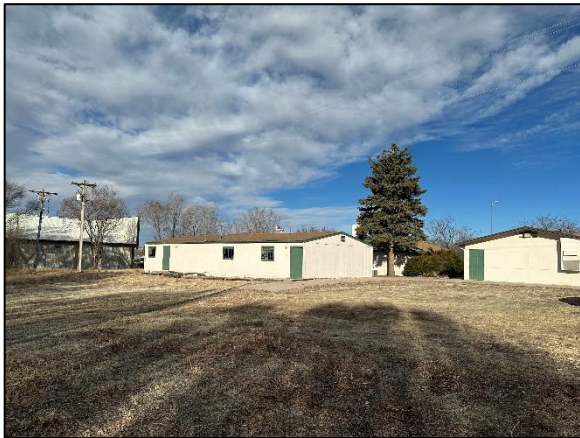
View looking northeast at the Subject
