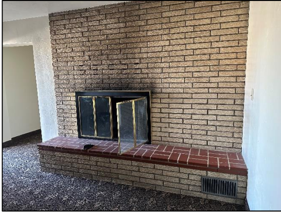
Lobby Fireplace (Building A)
