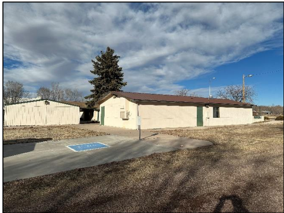
View looking north at Buildings B and C
