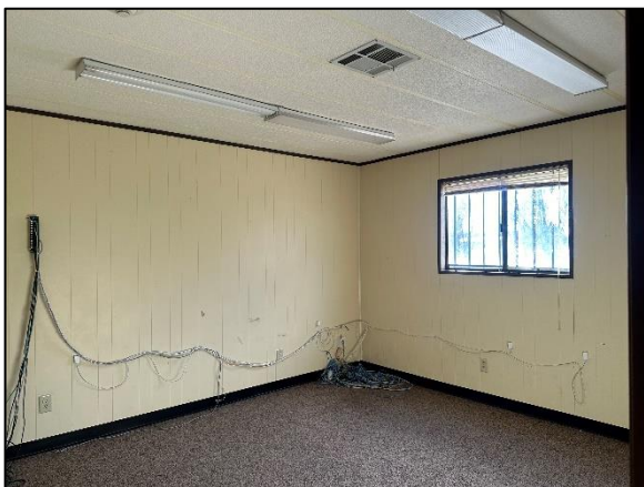
Interior View (Building B)
