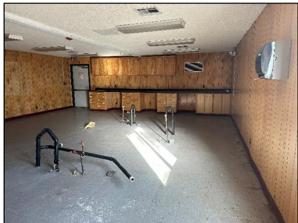
Interior View (Building C)
