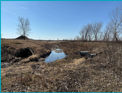
Existing Outfall looking south
