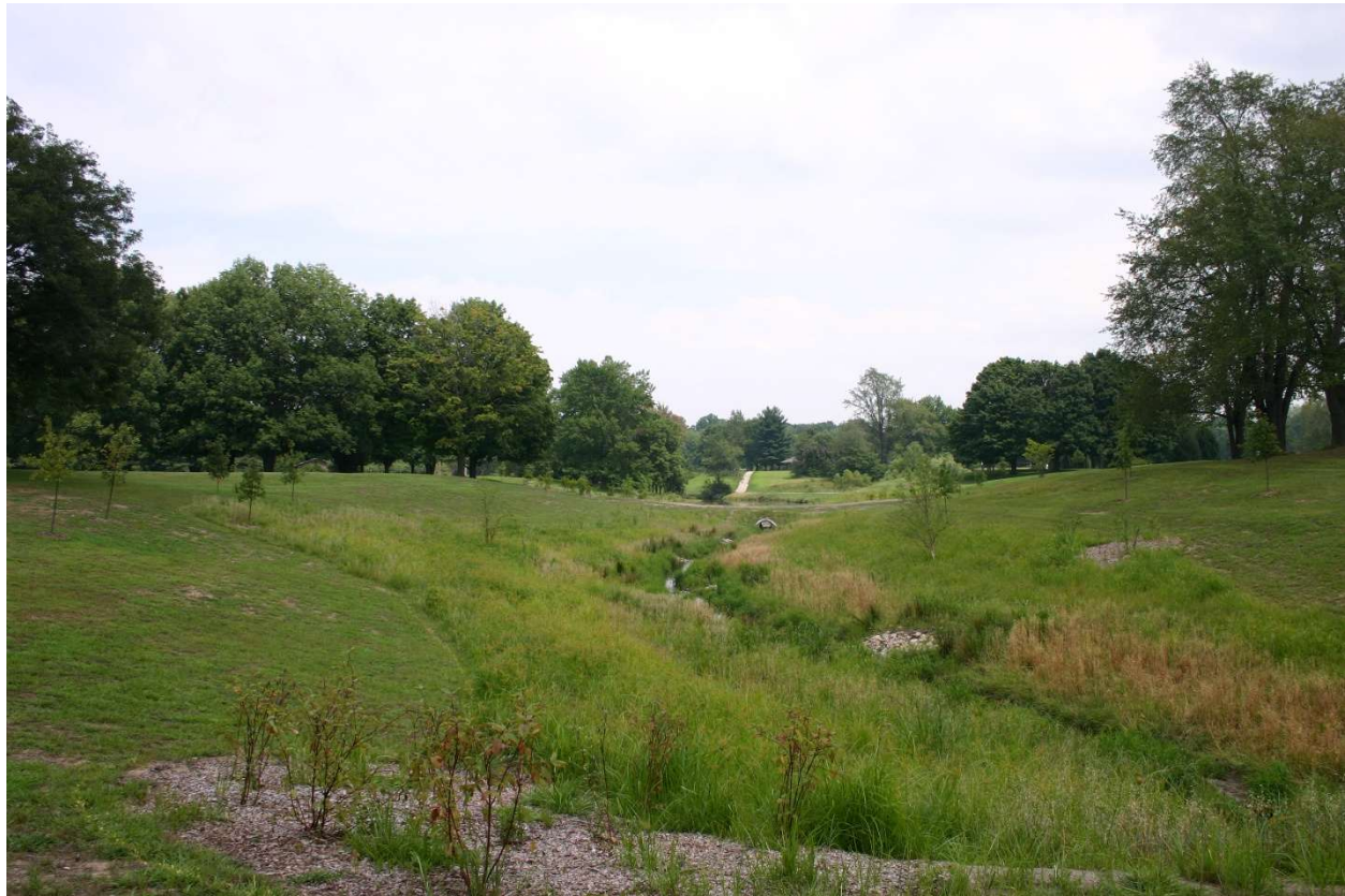
Figure 9: Examples of Vegetated Swales
