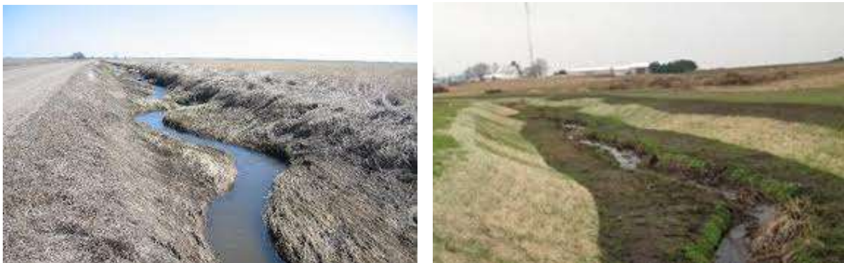
Figure 4: Examples of Two-Stage Ditches with Meandered Main Channel (Images from Minnesota Two-Stage Drainage Ditch Fact Sheet)
