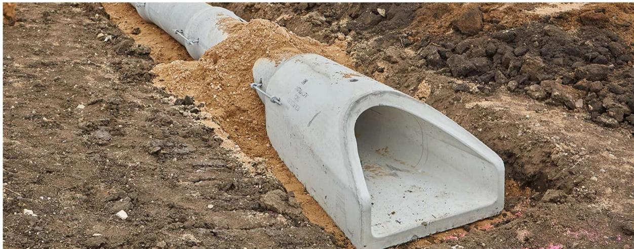
Figure 7: Concrete pipe with apron (Image from County Materials Corporation; https://www.countymaterials.com/news/precast-end-treatments )
