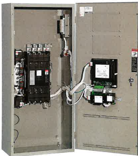
Fig. 16: ASCO 3ADTS/3NDTS 400 Amps Type 1 Enclosure
