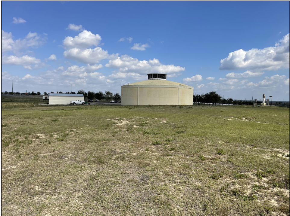
Figure C-2. Hickory Walk WTP Ground Storage Tank
