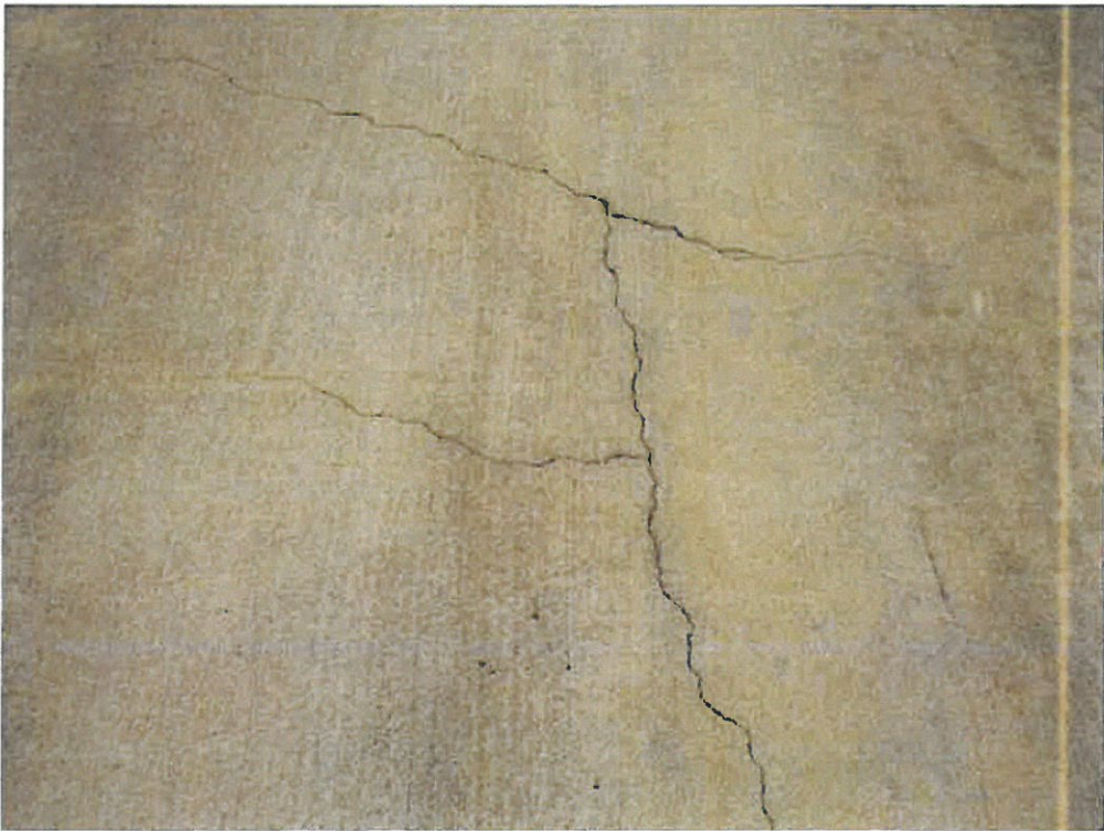
Cracking and Staining on Roof
