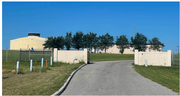
HICKORY WALK Water Plant
