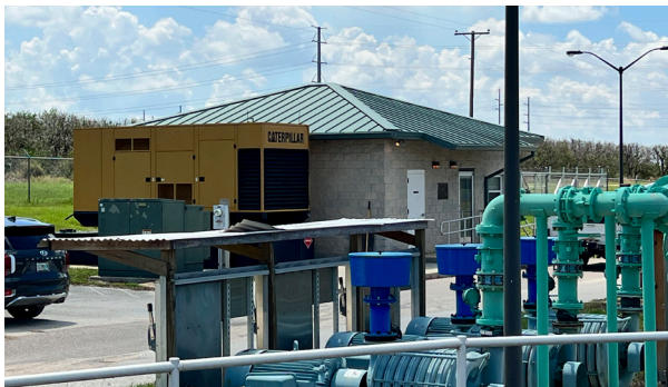
WWTF OPERATIONS office
