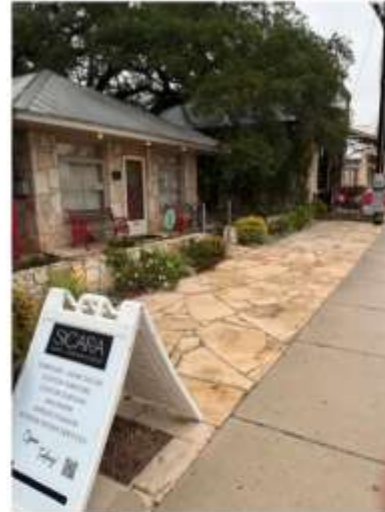
Flagstone Paving @ Mercer St
