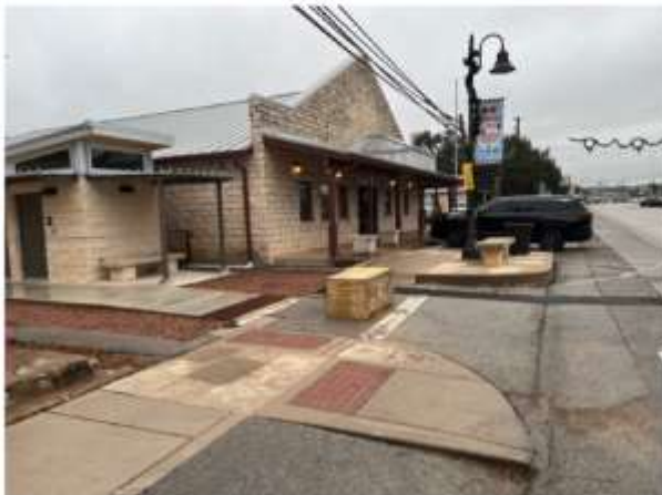
Existing Mercer Street Frontage
