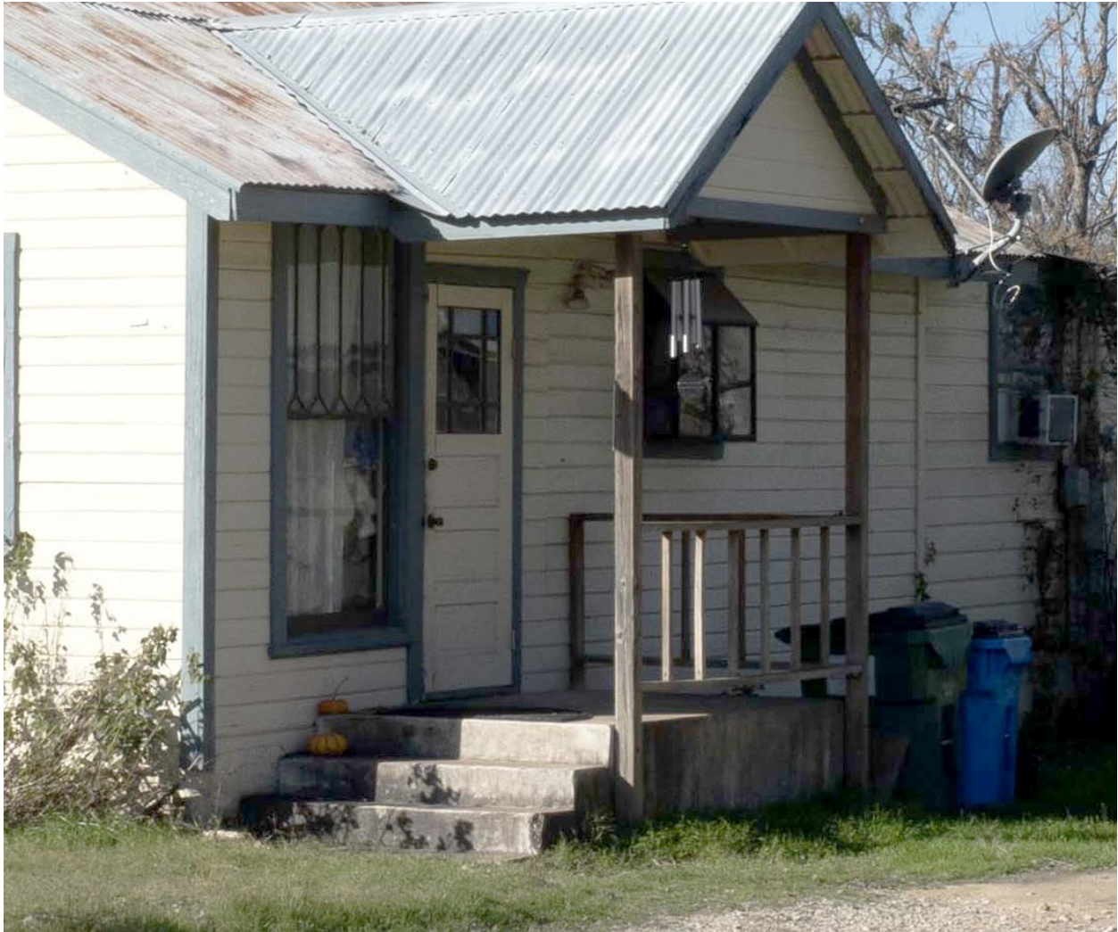
251 Old Fitzhugh Road: “detail of historic window”. Images from Post Oak Preservation, Old Fitzhugh Road Historic Resources Survey, 2024.
